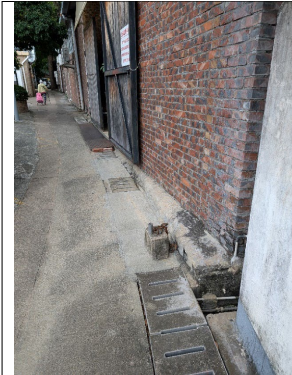
Plate 7 – Existing 225mm channel running along the eastern boundary of the Application Site flowing to the north.
